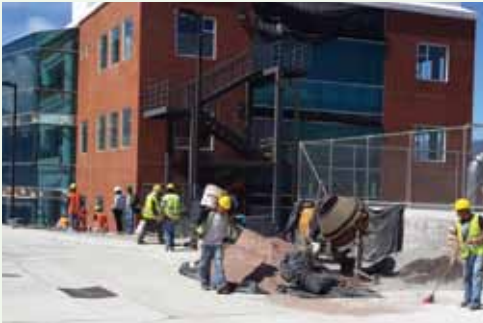
UNOPS construction at the IGSS Regional Hospital of Quetzaltenango, Guatemala. Photo: ©UNOPS
